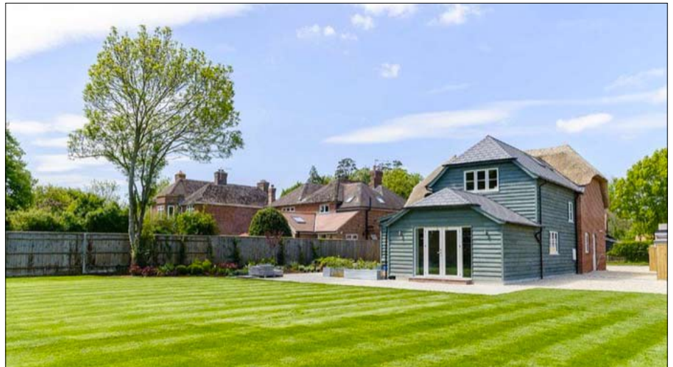
A hemp-based “eco-house” by Greencore Construction, UK. Asking price: €1.85 million ($2 million USD).
